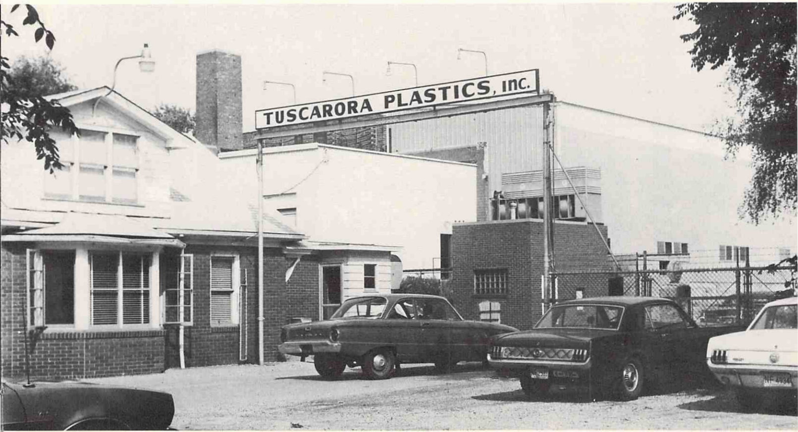
"Foremost in packaging" is Tuscarora Plastics, 701 S. Vermillion. The custom molders of expandable polystyrene have a very well equipped design and engineering department. There are 5 other Tuscarora Plants located in Ohio, Pennsylvania, Tennessee, New York and North Carolina. 815/672-2118
